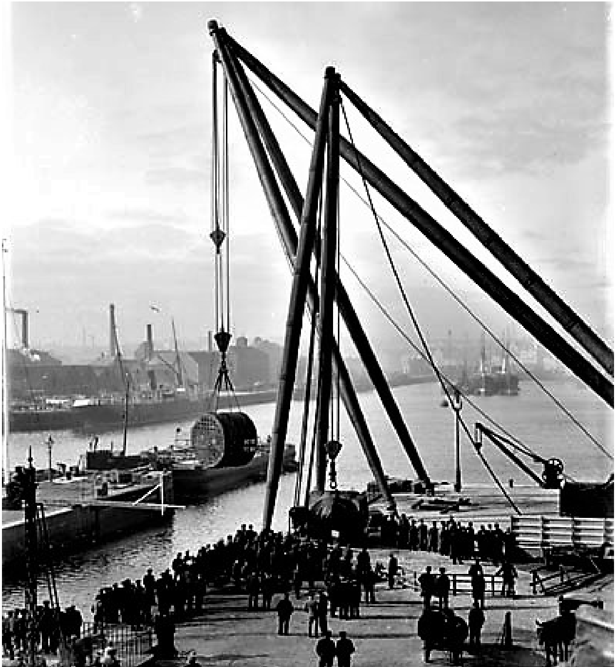
© http://www.abdn.ac.uk/historic/harbour/harb_single.php?harb_id=AHB2200 The newly installed 100-ton shear poles under load test in 1910 using a Scotch boiler filled with water.
