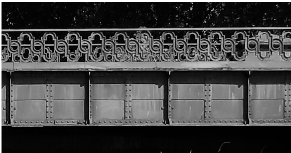
Bishops Mill Bridge, Elgin showing rivets and elaborately cast railings.
