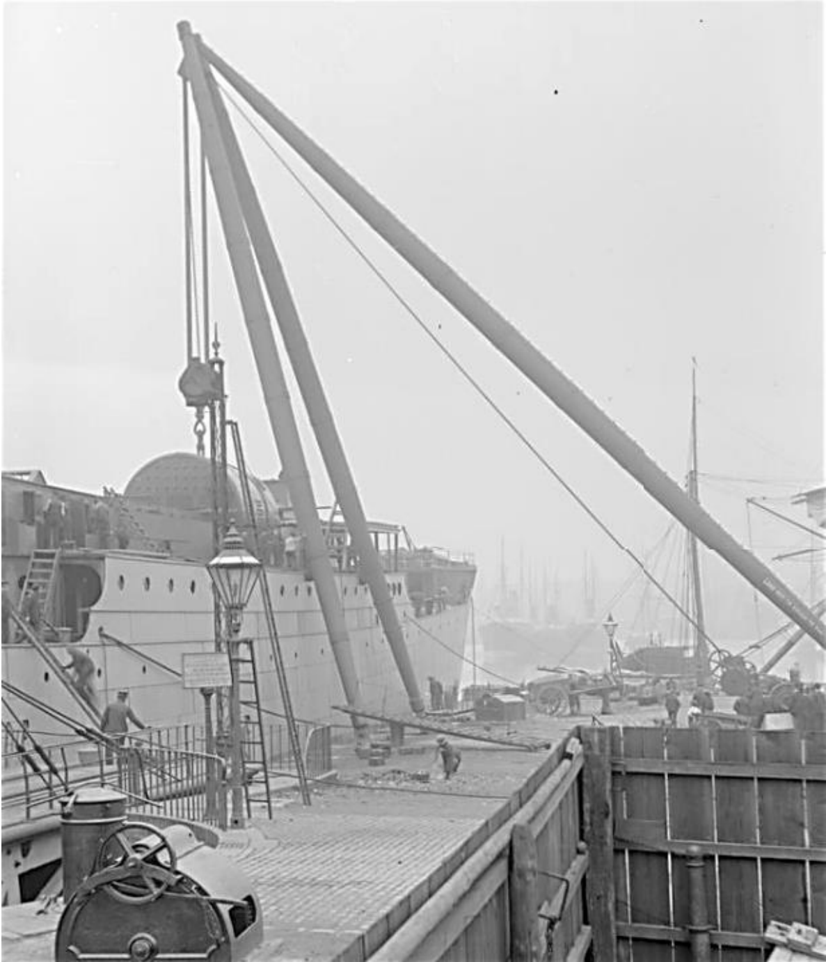
80-ton Shear Poles , lifting boiler onboard a vessel, pre-1910. Possibly a Rennie liner. (Photographer unknown, courtesy of University of Aberdeen / Aberdeen Harbour Board).
