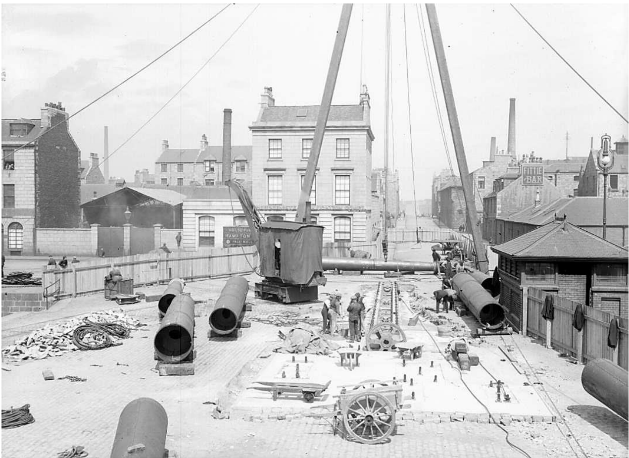
Assembly and erection of the 100-ton Shear Poles , 1910. (Photographer unknown, courtesy of University of Aberdeen / Aberdeen Harbour Board).
