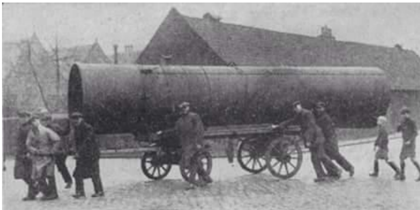
Seven men manually transporting a funnel for a steamer to the Shear Poles for erection. (Photographer unknown).
