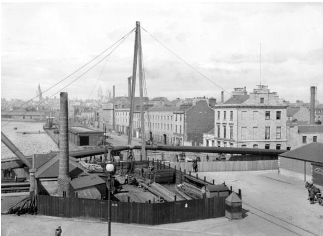
Erection of the 100-ton Shear Poles in 1910, using temporary wooden shear poles . 80-ton Shear Poles winch-house and chimney in the foreground left. (Photographer unknown).
