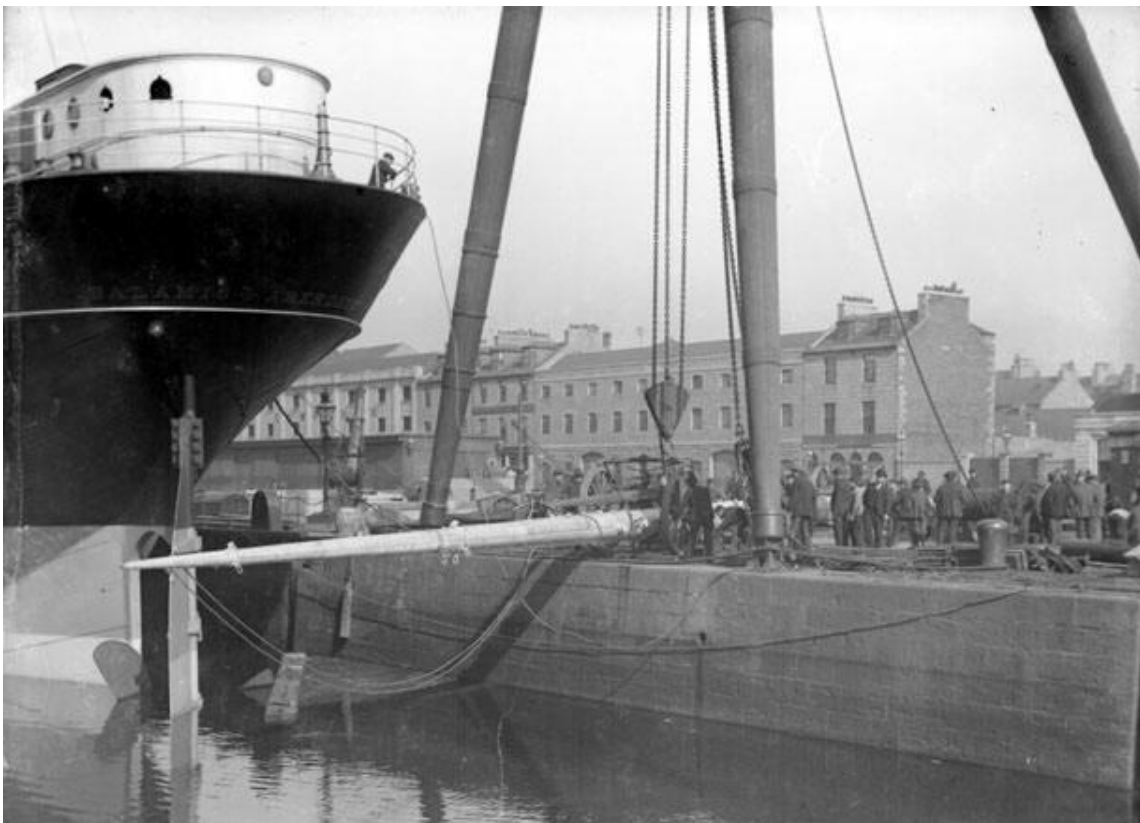
About to erect a mast on s.s. 'Salamis' (4,508 tons) in 1899 using the 80-ton Shear Poles . (Photographer unknown, courtesy of University of Aberdeen / Aberdeen Harbour Board).
