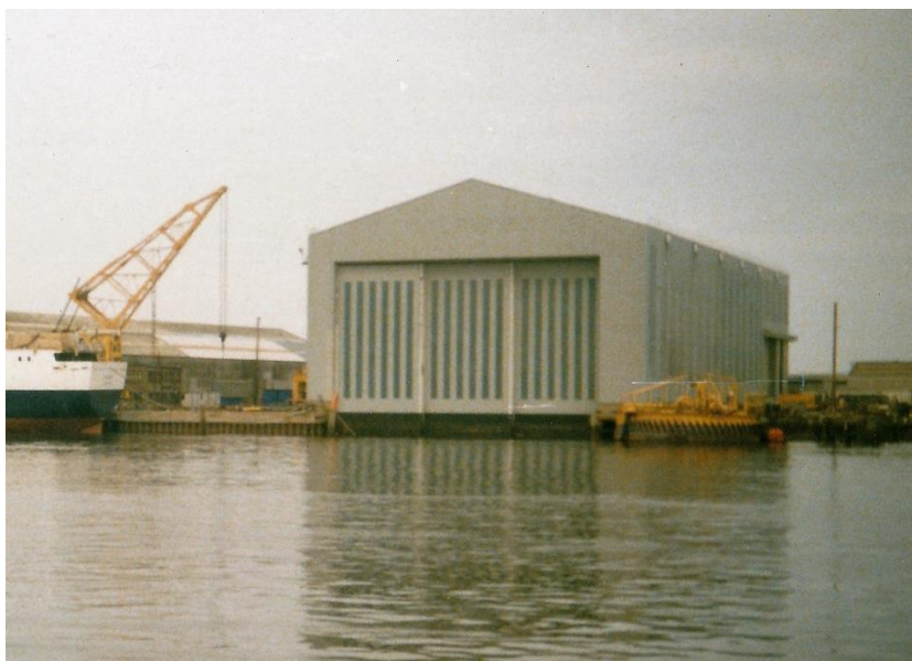
Hall Russell Ltd, Building Hall and 65-ton crane, 1990. (S. Bruce).
