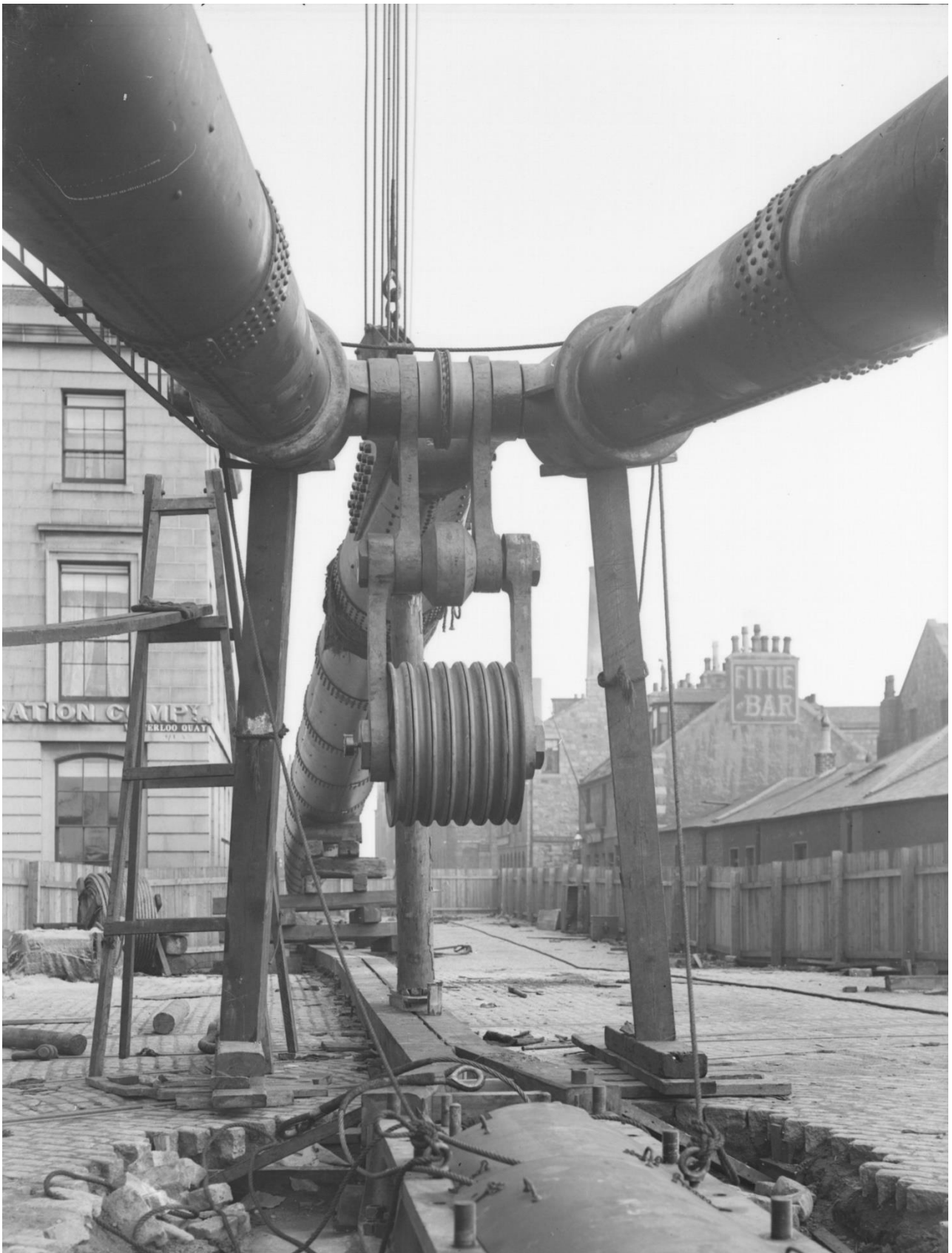
Seven sheaves Crown Block of the 100-ton Shear Poles. (Courtesy of University of Aberdeen / Aberdeen Harbour Board).
