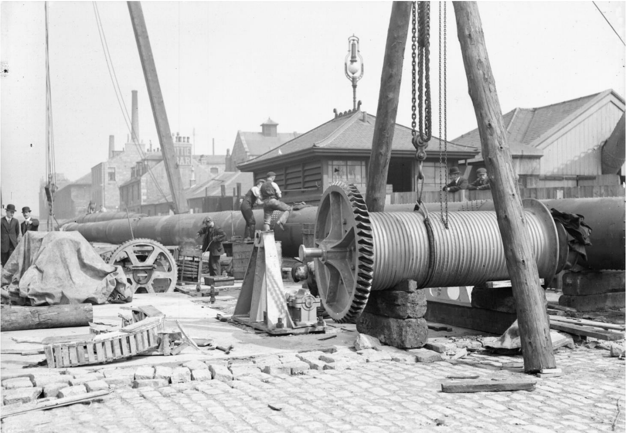
100-ton Shear Poles Wire winch drum. (Photographer unknown, courtesy of University of Aberdeen / Aberdeen Harbour Board).
