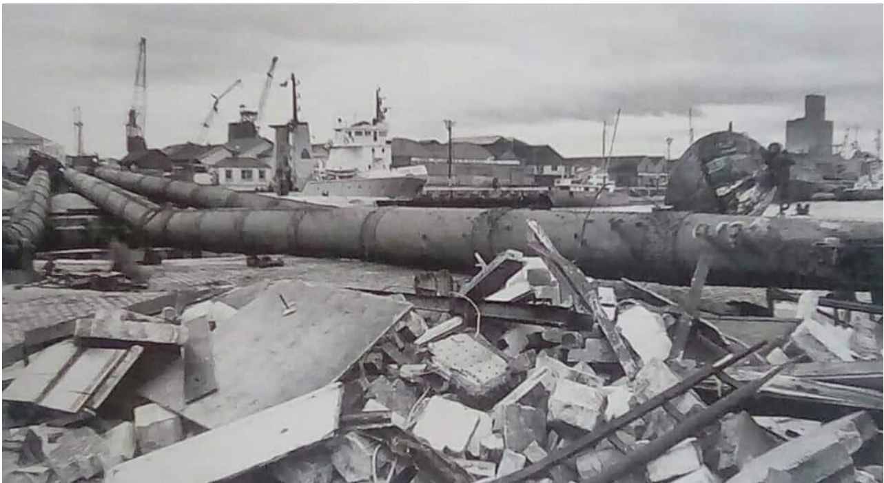
Demolition of the 100-ton Shear Poles in 1975. (Aberdeen Journals).
