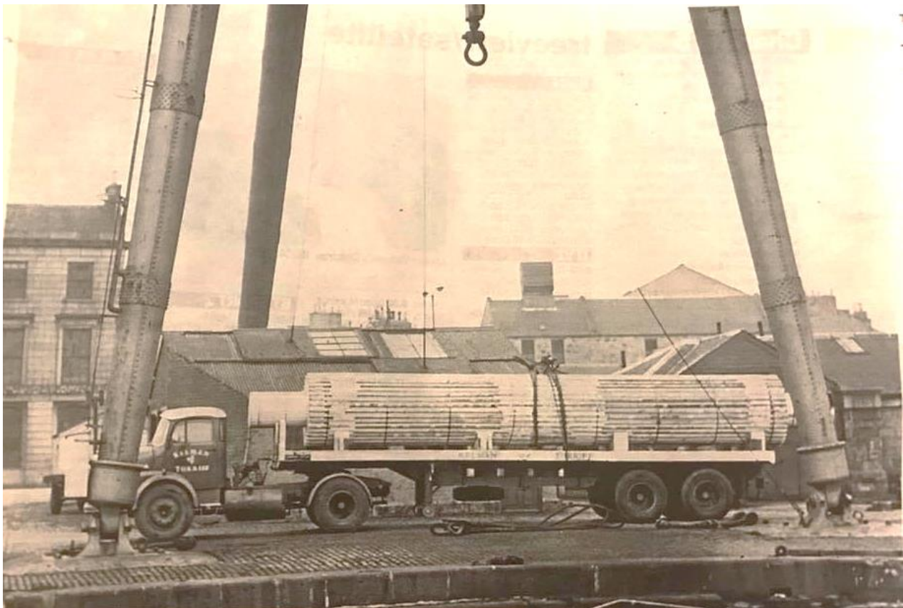
100-ton Shear Poles prepares for a heavy lift in 1966. (Aberdeen Journals).
