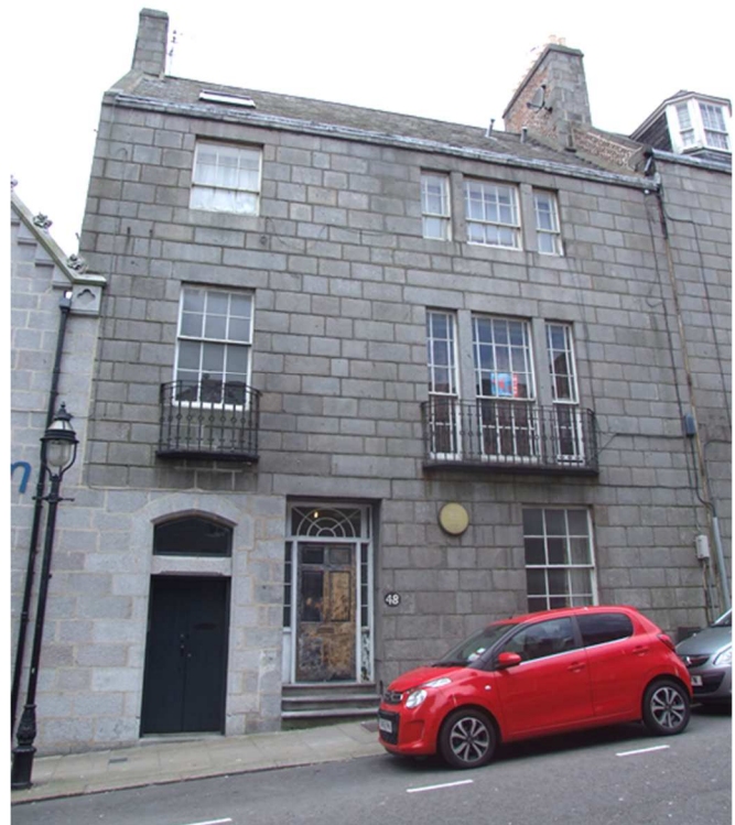
Former offices of J. T. Rennie, No. 48 Marischal Street, Aberdeen. (S. Bruce).
