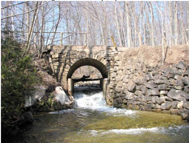
View north to south elevation (downstream).
