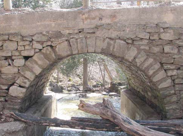
Stone arch of bridge upstream side..
