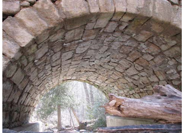
View southward to underside of the stone arch.
