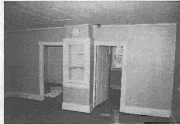
21. Bedroom doors and chimney shaft.
