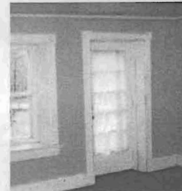
25. Detail showing thick walls at front door and window.
