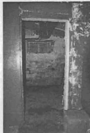
16. Door to cold cellar from utility area.
