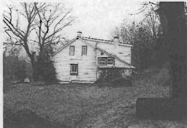
7. East elevation showing dormer and lower utility/ cold cellar area.
