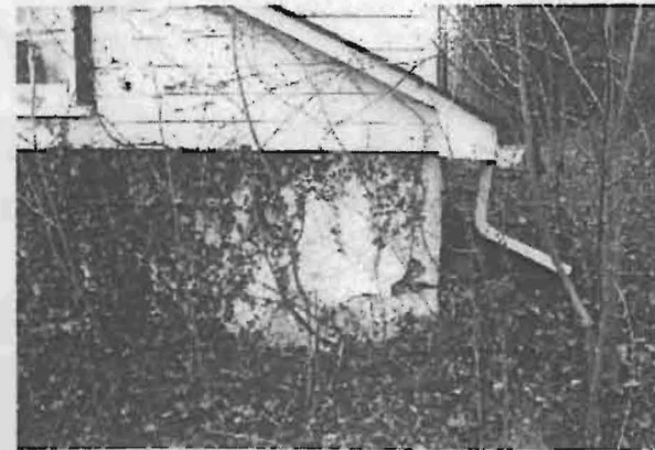
8. Close up of the utility/cold cellar wall. Plaster on stone.
