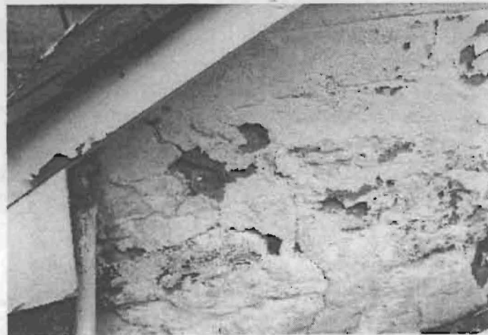
10. Close-up of the cold cellar wall showing a relatively thick layer of plaster over rubble stone. The plaster has a reddish colour indicating a local sand was used.
