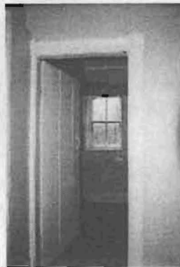
22. South-west bedroom window. Note plank door and latchset.
