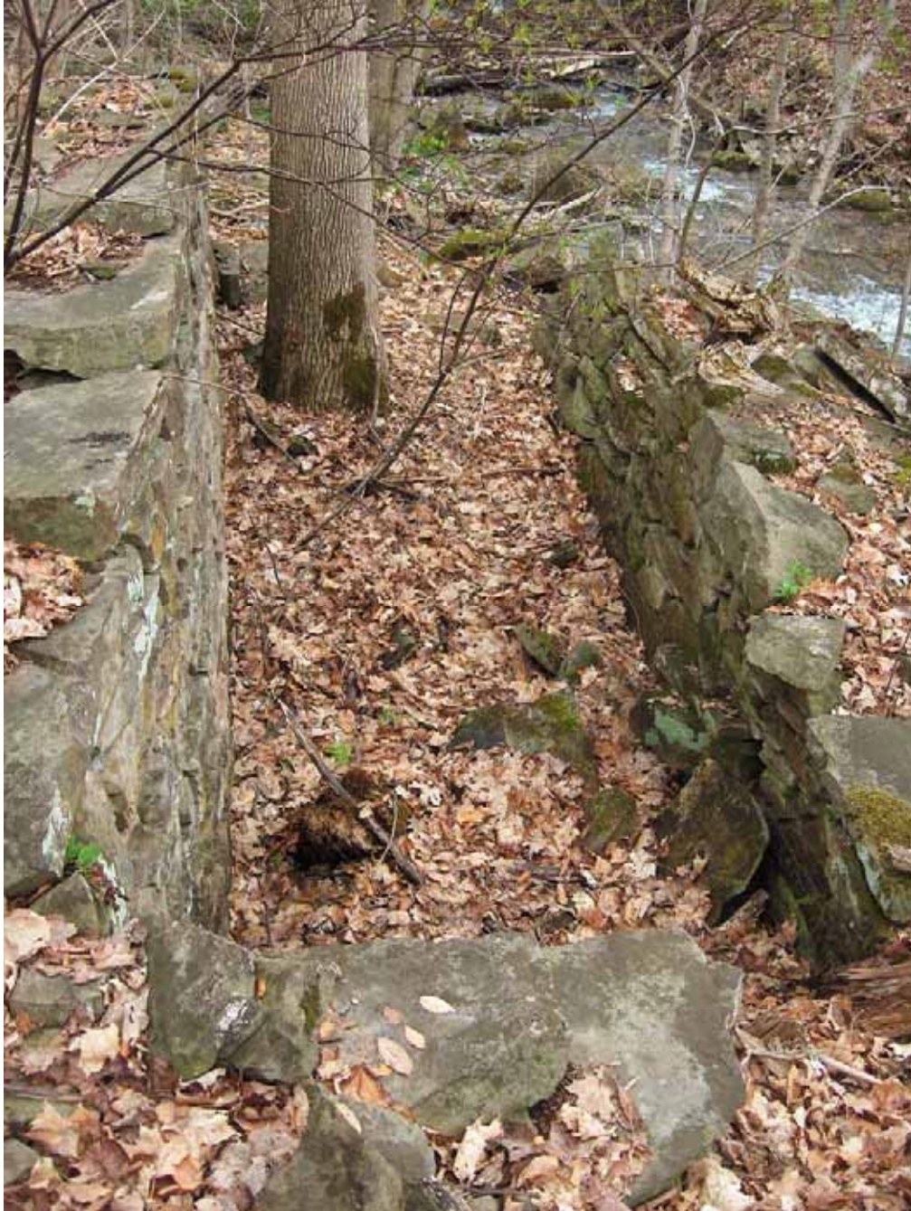
4.18 View down into wheel pit. The west wall of the stone foundation has suffered more outward collapse, possibly due to floodwaters from the creek. It is believed to have been the same height as the east wall, so that the axle for the millwheel could be supported by both walls. The pit may extend several feet below the level of the leaves, which would create enough height for an overshoot wheel at least 14 feet in diameter and 4 feet wide. This is a large wheel which could provide approximately 25 horsepower to run a grist mill. The area to the east of the wall has several large stones that appear to be placed and leveled to carry the timbers which supported the timber framed mill building.
