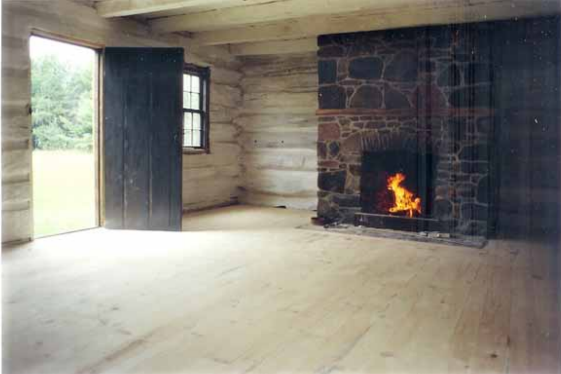
Interior of another example, the reconstructed Puterbaugh Log House, whitewash on walls & ceiling.
