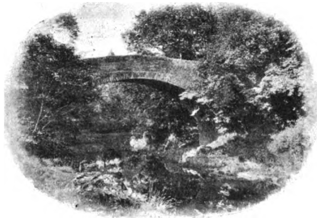
HORNS HOLE BRIDGE.
