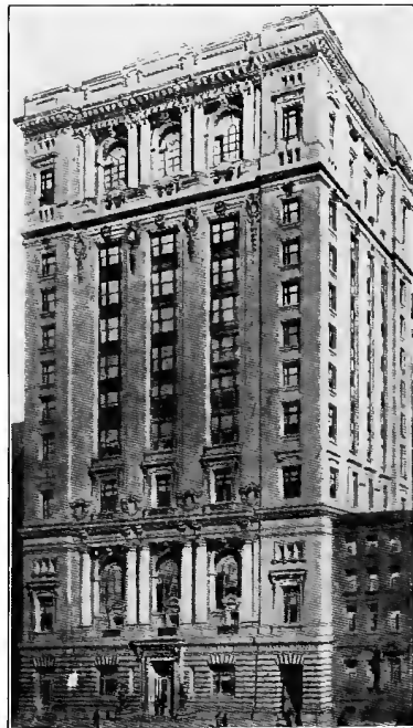
United Engineering Societies Building. New York
