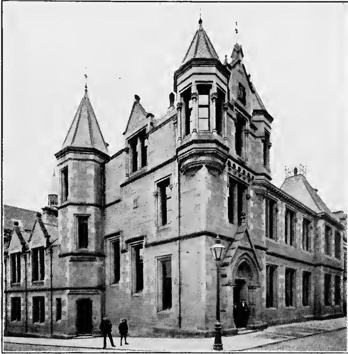
Carnegie Free Library, Dunfermline. This was the first of all the library buildings erected by Mr. Carnegie. The cornerstone was laid by Mrs. Margaret Morrison Carnegie, Mr. Carnegie's mother, July 27, 1881. The Library was formally opened by Lord Rosebery, August 29, 1883.
