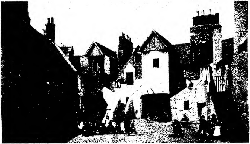
FIG. 5.—Surviving court in Canongate, with outside stairs, etc.
