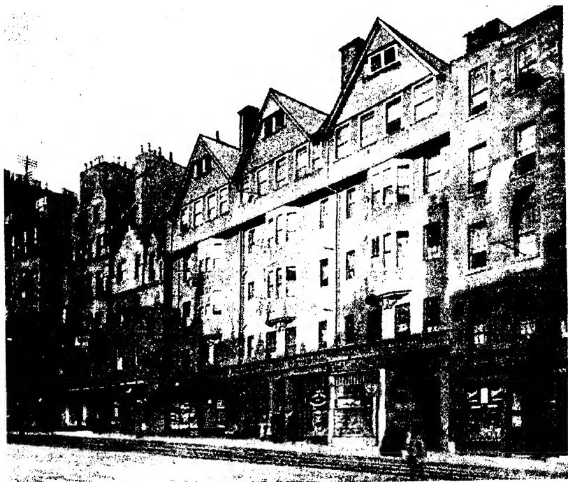
FIG. 29.—An improved tenement house (1892) in Lawnmarket (Upper High Street), Edinburgh.
