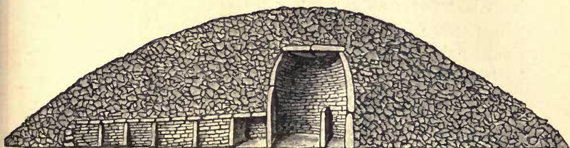
Fig. 250.—Section along Passage and through the Chamber of Chambered Cairn at Camster, Caithness (75 feet in diameter).
