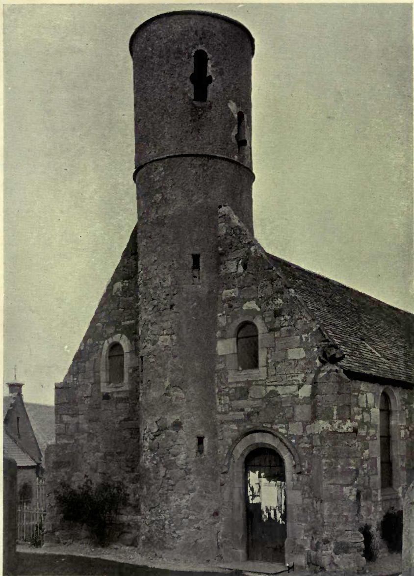
COCKBURNSPATH CHURCH: TOWER
