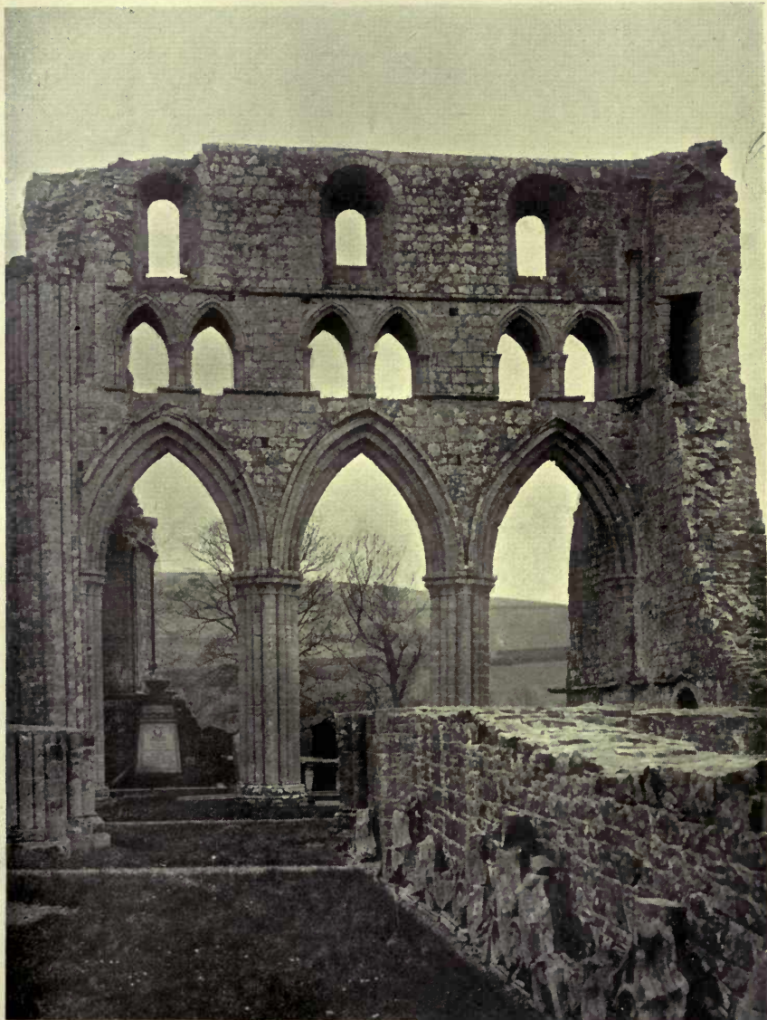
DUNDRENNAN ABBEY: SOUTH TRANSEPT
