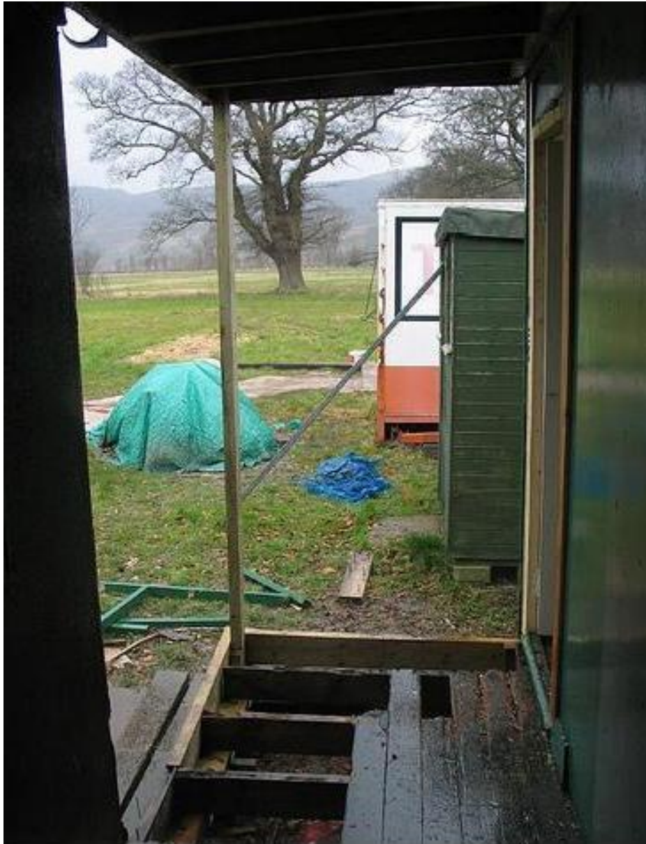
Springtime repairs at Meiklewood Pavilion
