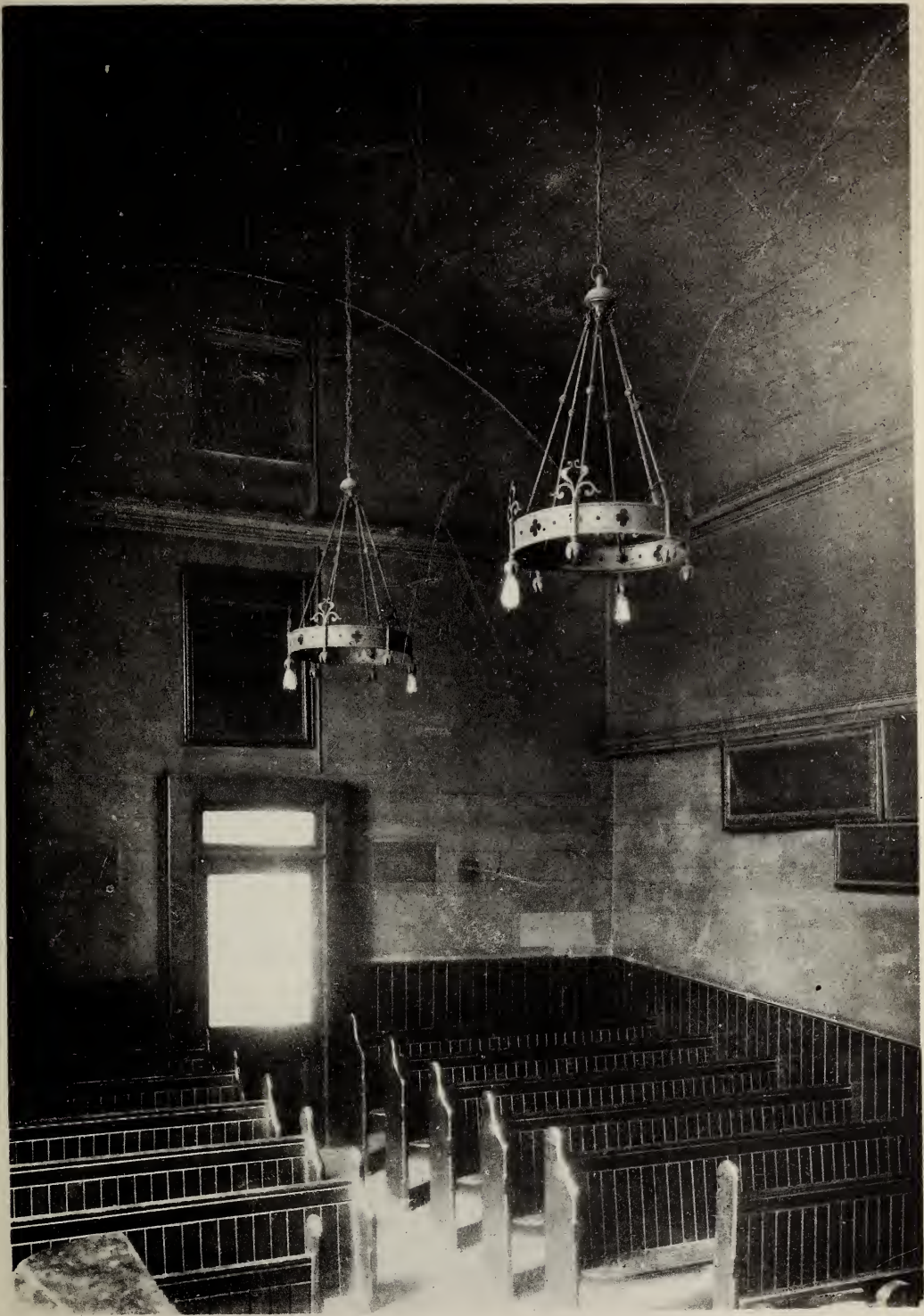
(FIG. 3) INTERIOR VIEW OF THE CHAPEL TO THE NORTH-WEST
