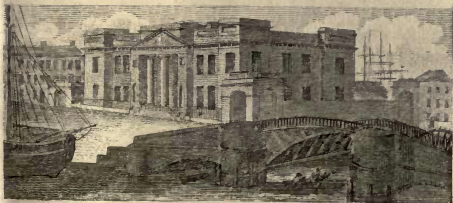
Custom House, Leith.
