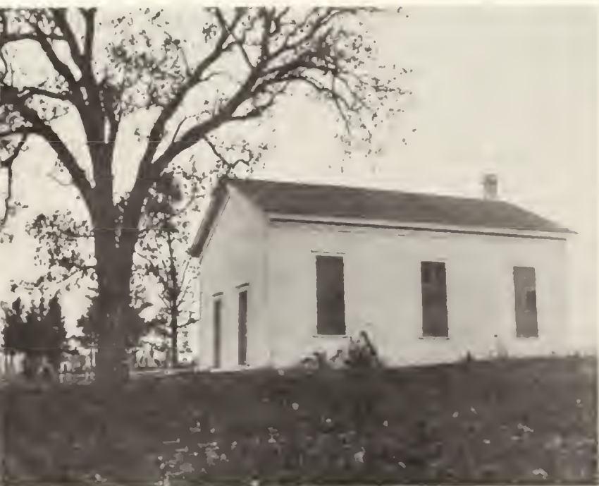
CENTER GROVE CONGREGATIONAL CHURCH AND CEMETARY TOWN OF CENTER, ROCK COUNTY, WISCONSIN
