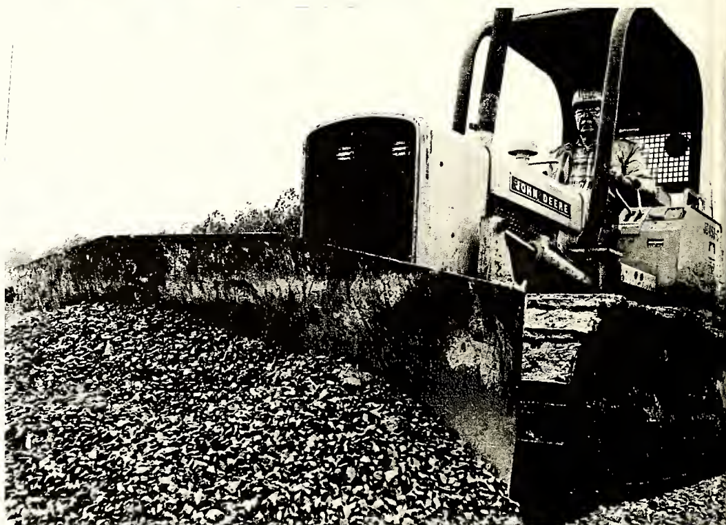
Red Neville at work on his company's demolition of the old Antioch Baptist Church 1973
