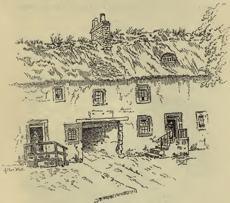
Old Houses, Newburgh.
