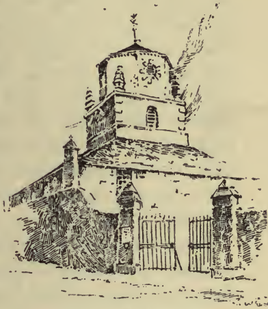
Burntisland Parish Church.
