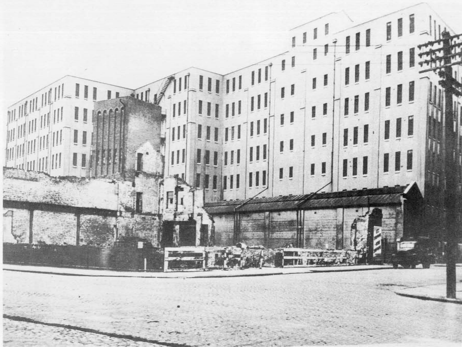
FIGURE 6.—Stanley Tobacco Warehouse Used by General Depot 14
