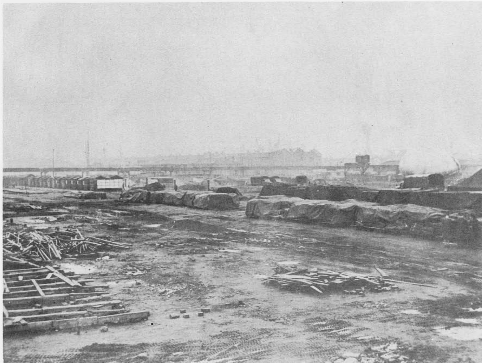
FIGURE 7.—Open Storage in Blitz Park
