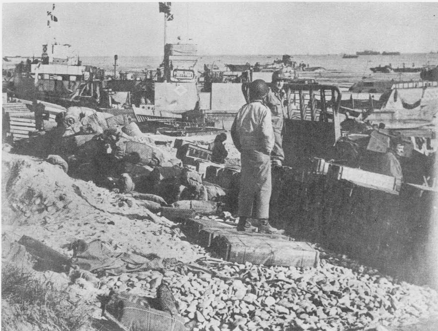
FIGURE 16.—Landing Supplies from Ships at the Edge of the Beach Flat
