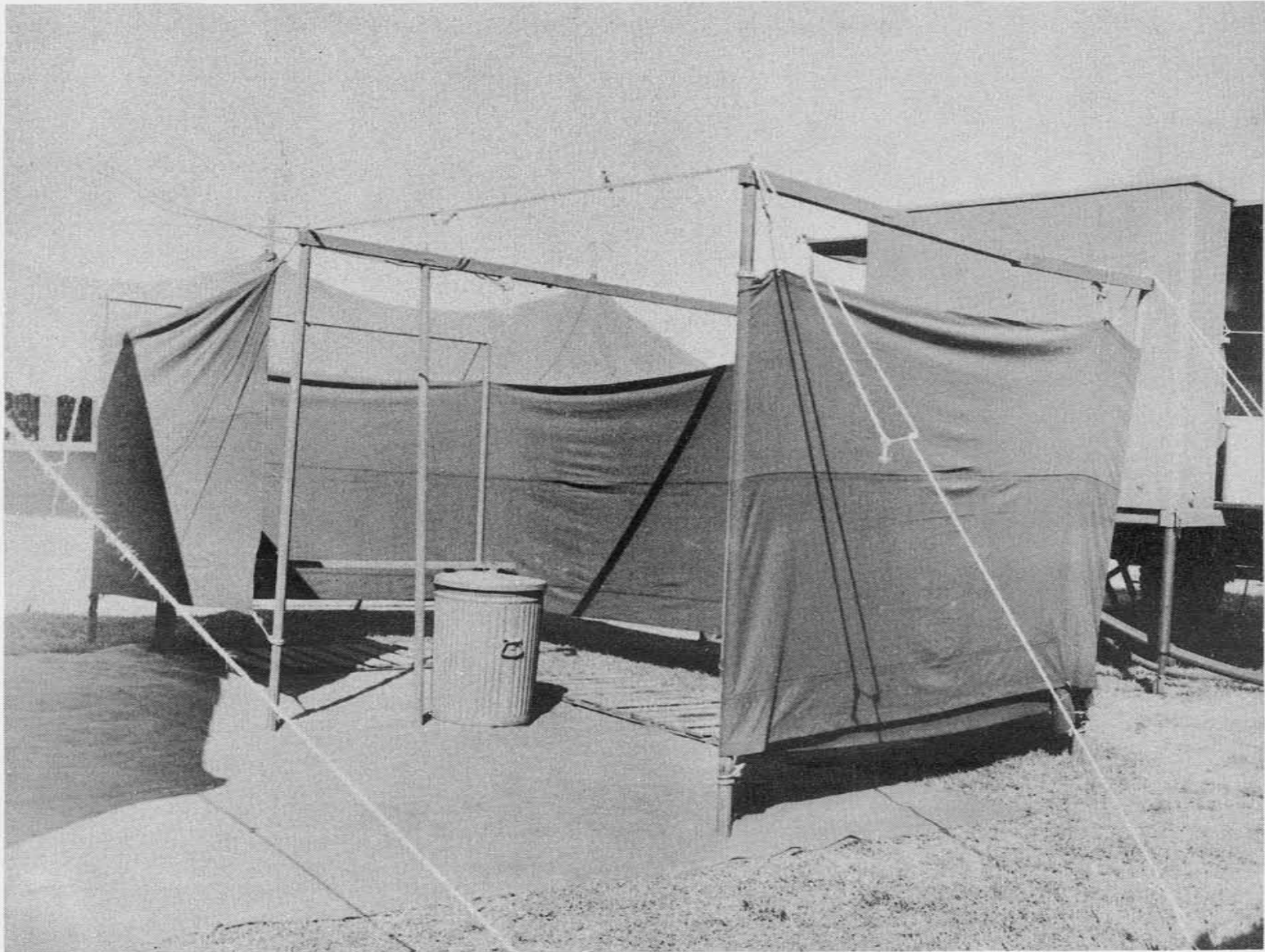
Figure 34.—Latrine Screen with One Section Omitted.
