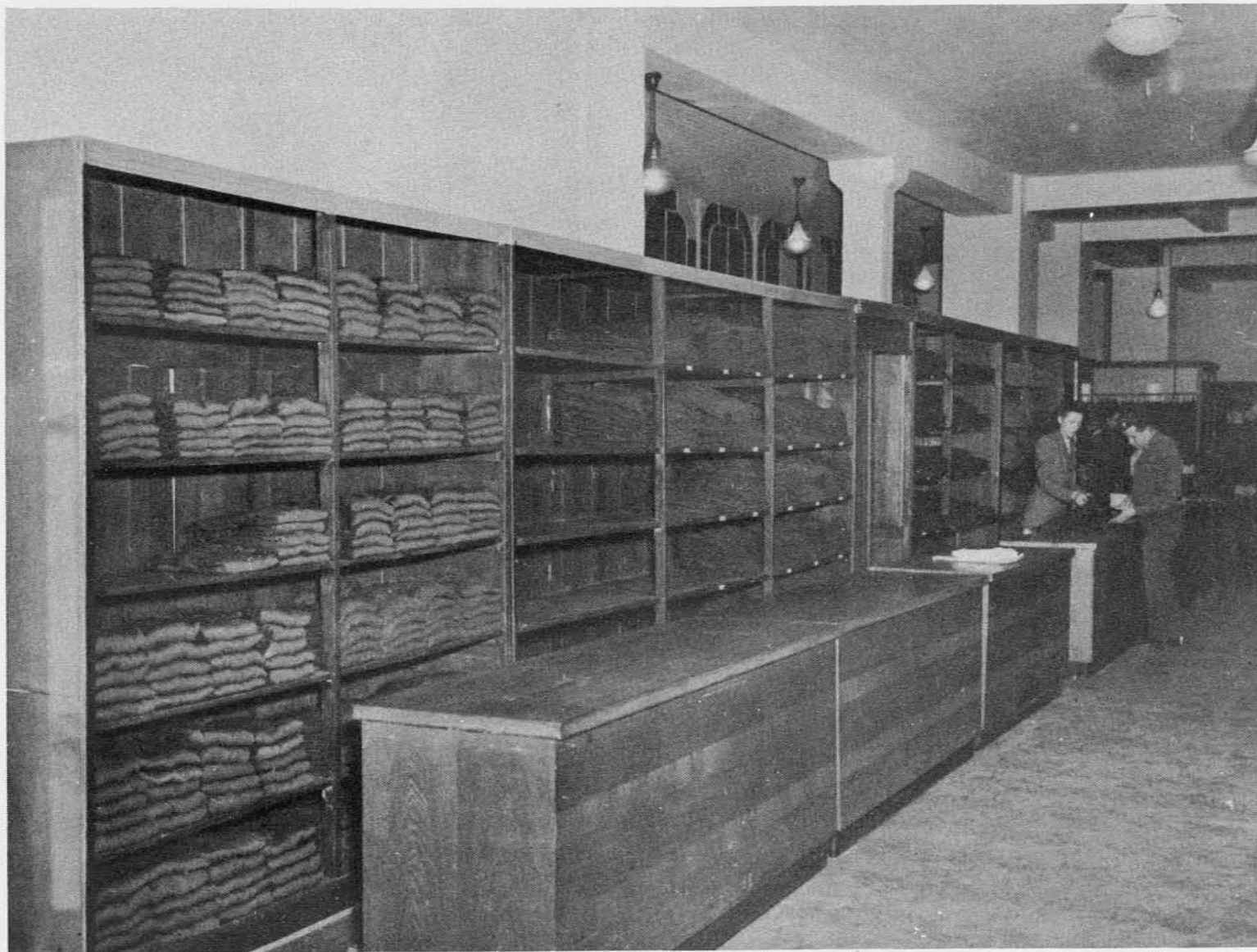
Figure 18.—Interior of the Berlin Sales Store.
