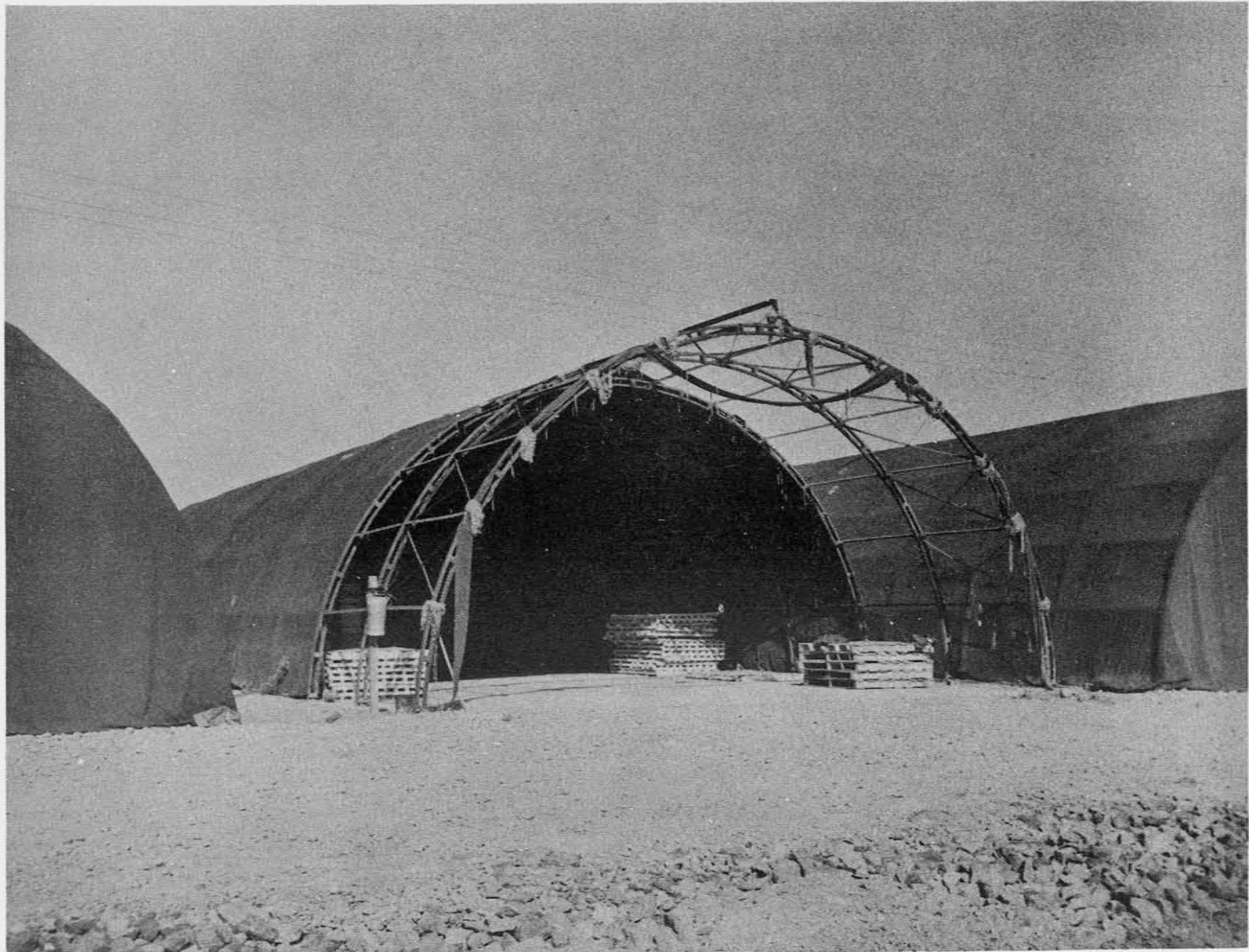
Figure 36.—Semi-Romney Huts under Construction on the Continent.
