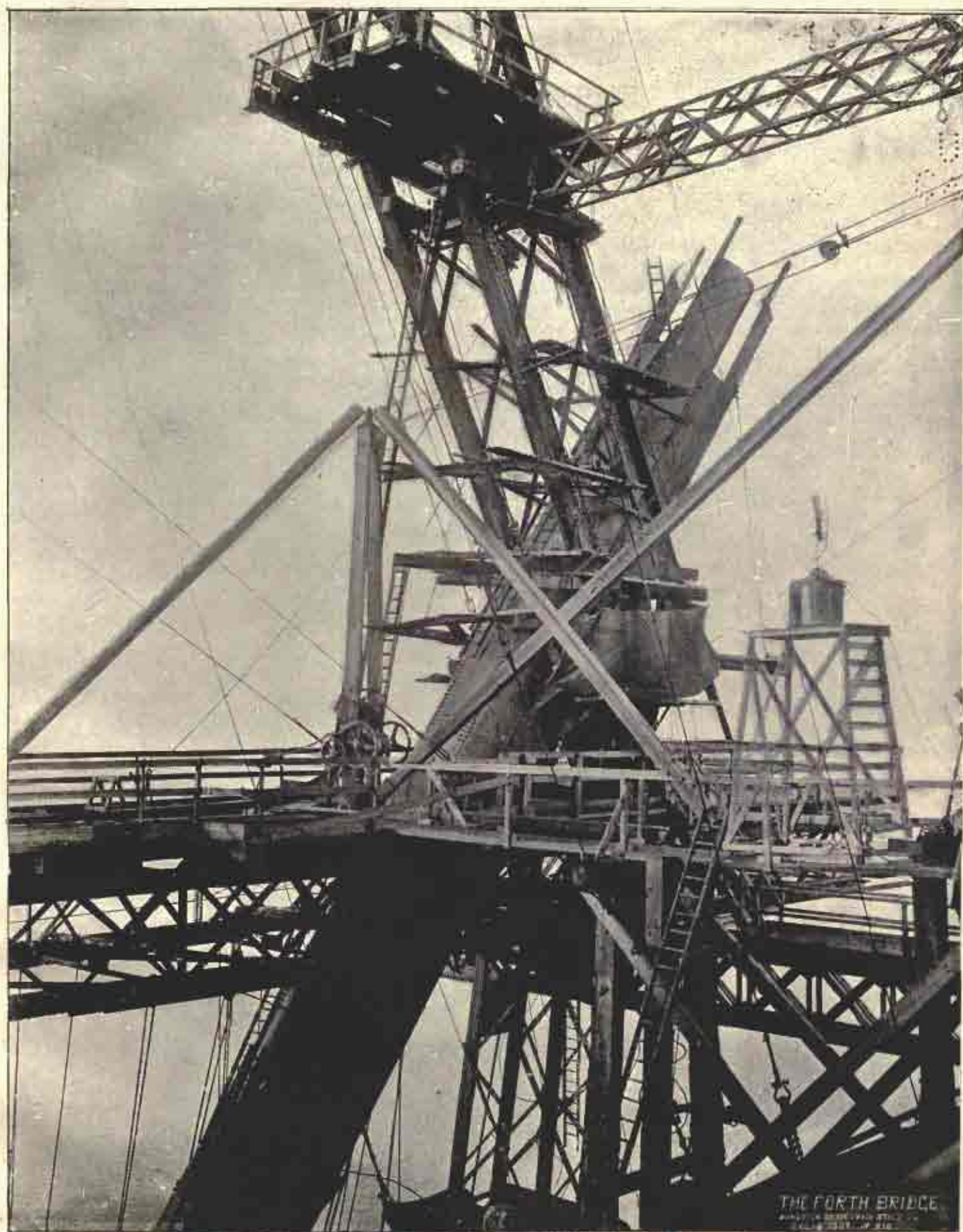
MAKING GOOD A CROSSING BETWEEN STRUTS AND TIES IN FIRST BAY OF CANTILEVERS.
