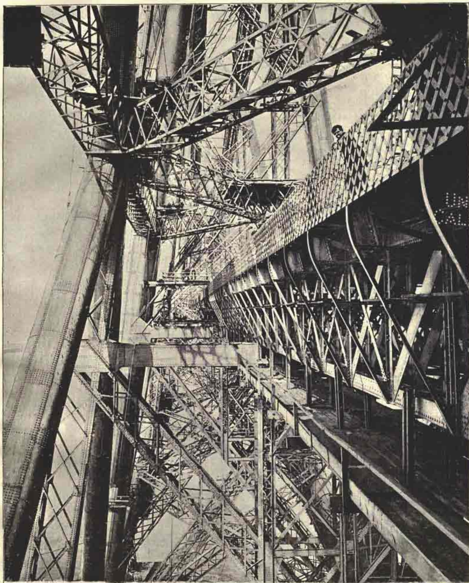
CENTRAL TOWER OF INCHGARVIE; INTERNAL VIADUCT GIRIERS AND WIND FENCE.
