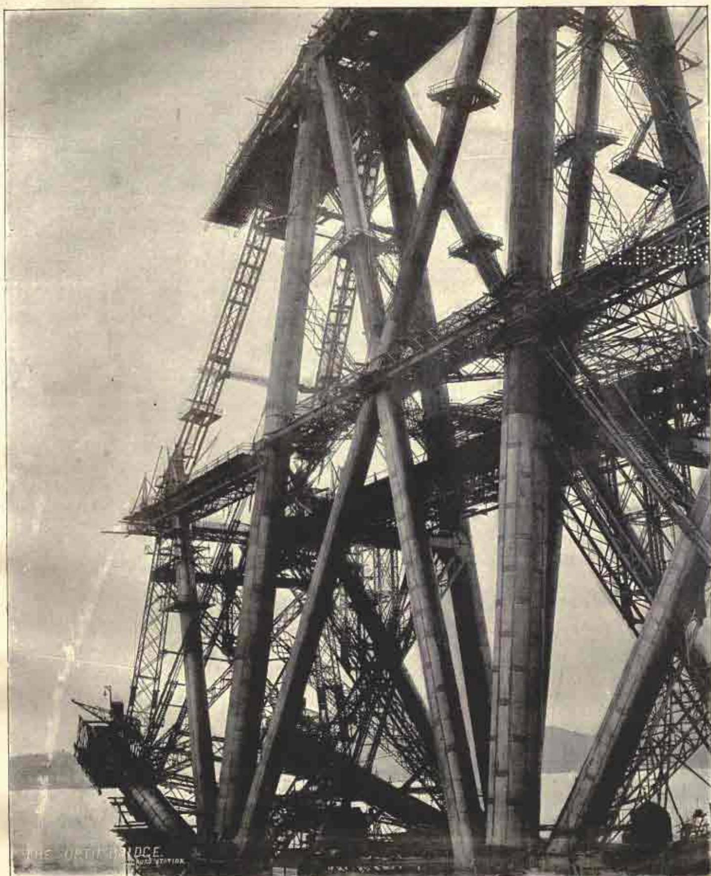
FIFTH PIER. CENTRAL TOWER AND LOWER HALF OF FIRST BAY IN FREE CANTILEVER.
