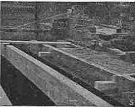
Fig. 5. Trimmers and trimming joist, showing tusk-tendon joint.
