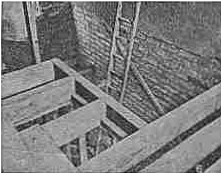
Fig. 6. Flooring and joist around a staircase well or opening.
