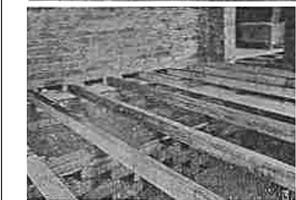
Fig. 2. Sleeper walls, showing damp course slates, upon which floor plate and joists are laid.
