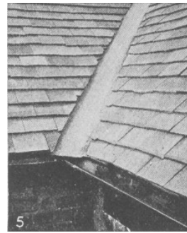
Fig. 5. Valley gutter, showing tiles cut back.
