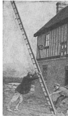
Ladder. Fig. 1. Correct positions when raising a ladder. Fig. 2. Method of lowering a ladder so that one man acts as a counterbalance to the weight borne by the man who holds it up.
