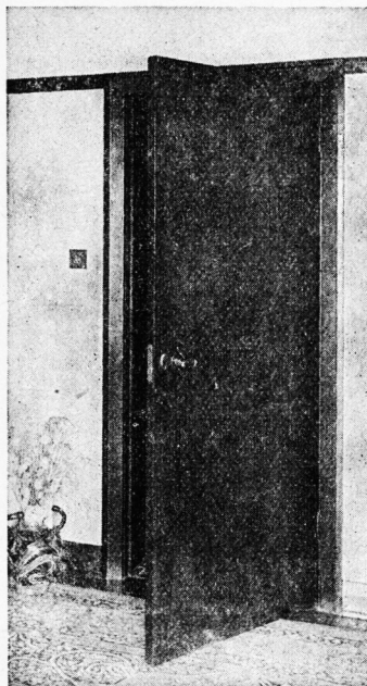
Plywood flush door for dining room; American walnut, with oak on the reverse side. Size, 2 ft. 8 in. by 6 ft. 6 in.
