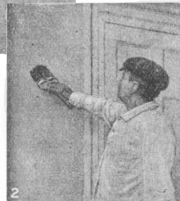
2. Correct way to apply distemper is by working at arm's length.
