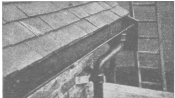
Gutter. Fig. 1. Down pipe swan-neck, and stop-end of an eaves gutter system.
