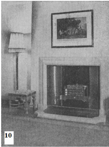
Fig. 10. A gas-coke grate. Quickly lit by gas, which is turned off when the fire is well alight burns evenly without smoke or soot.
