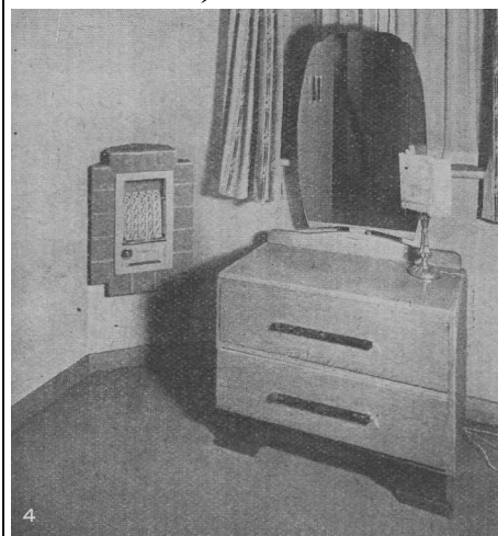
Fig. 3. A built-in gas fire suitable for a modern sitting room or dining room. The self-lighting mechanism is concealed in the base of the fire. (British Commercial Gas Association)
