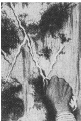
Graining: Stages in marbling wood. Left, wiping the veins with a thumb rag. Right, completing with a feather dipped in colour.
