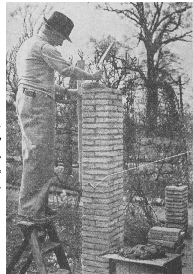
How to build pergola piers of thin rustic bricks; careful plumbing course by course is important to ensure a truly vertical pier.
