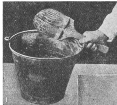
2. Correct way to apply distemper is by working at arm's length.
