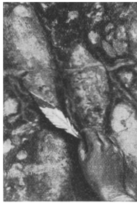
Graining: Stages in marbling wood. Left, wiping the veins with a thumb rag. Right, completing with a feather dipped in colour.
