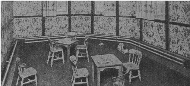
Fig. 9. "Unity" Tubular System installed in a nursery school. Heating tubes are attached by brackets to the skirting boards and the system operates by low temperature radiation.
