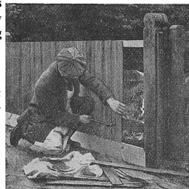
Fence. Fig. 1. Repairing a cleft oak pale fence with new gravel boards.
