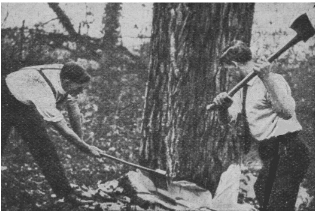
Axe. How to hold to obtain the correct swing in felling a tree.
