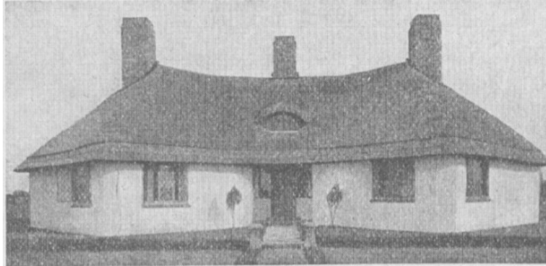
Bungalow. Fig. 3. Bungalow at Beaulieu, Hants. The walls are made of pisé-de-terre.
