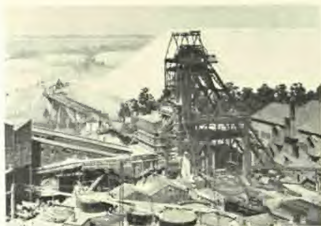
61. Crown Mines, Johannesburg, showing the headgear of the main shaft and the reduction plant in the foreground and the dumps of waste material in the background. Crown Mines, with working levels over 9,000 feet below the surface, are the deepest mines in the world and up to the end of 1955 had yielded over 40 million fine ounces of gold; 25 per cent more than their nearest rival.
