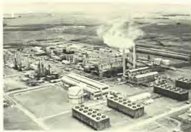
66. The Sasol oil-from-coal plant. In the foreground are the cooling towers. Behind, left, is the Oxygen Plant and then the American Catalytic Synthesis Section and the Products Recovery Section. Behind, right, are the power station, the Gasification Plant and the German Catalytic Synthesis and Recovery Sections. In the background are the By-Products Section and the Storage Tanks.
