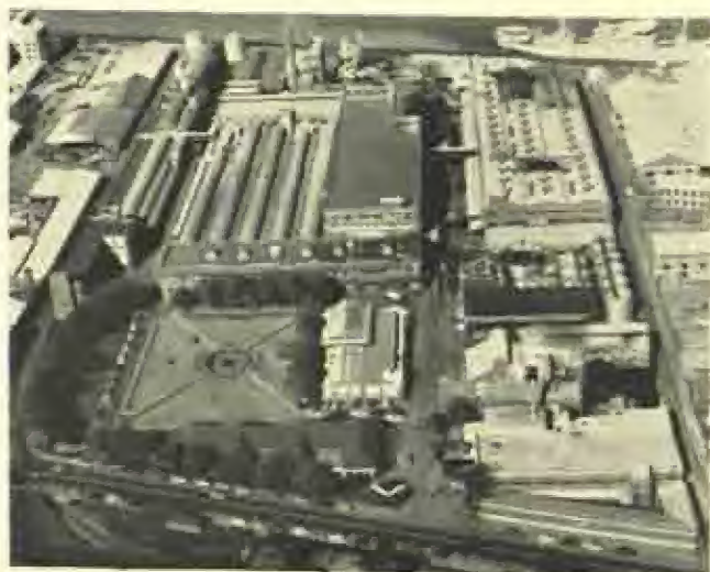
70. The Modderfontein explosives factory. In the foreground are the new ammonia and nitric acid plants. Parts of the explosives area can be seen on the right screened by trees. Centre is one of the five dams constructed along the Modderfontein river (tributary of the Jukskei) to provide water. Land irrigated for vegetables occurs below the dam on the far bank of the stream. Behind the dam are two housing estates.
