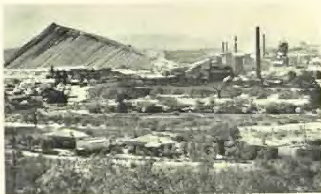
61. Crown Mines, Johannesburg, showing the headgear of the main shaft and the reduction plant in the foreground and the dumps of waste material in the background. Crown Mines, with working levels over 9,000 feet below the surface, are the deepest mines in the world and up to the end of 1955 had yielded over 40 million fine ounces of gold; 25 per cent more than their nearest rival.
