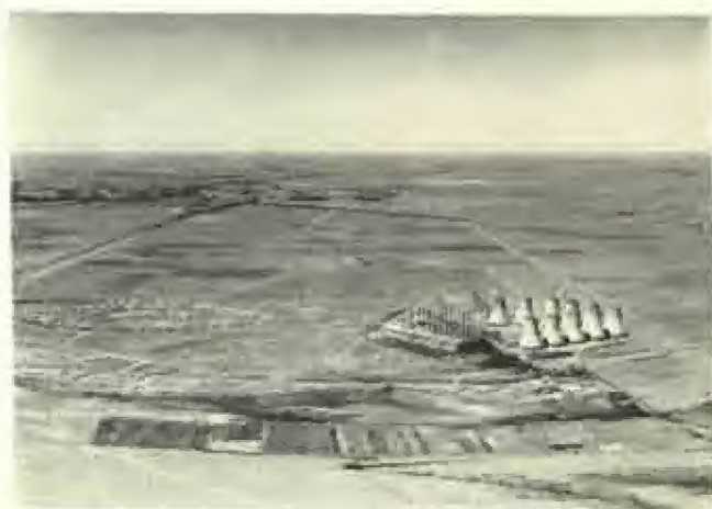
64. Typical Witbank colliery. The coal seams are approached not by a shaft but by a cutting seen disappearing into the ground (centre right).
