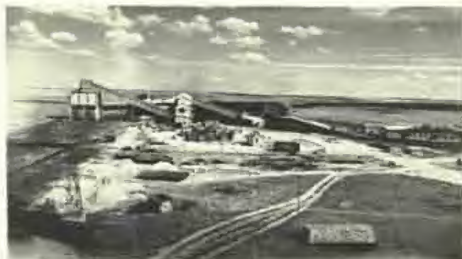
64. Typical Witbank colliery. The coal seams are approached not by a shaft but by a cutting seen disappearing into the ground (centre right).
