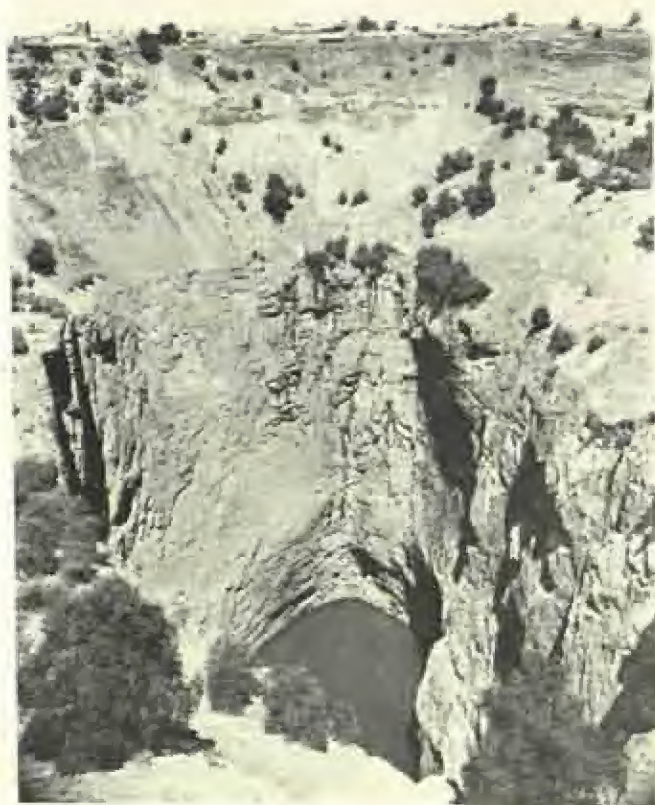
59. The Big Hole at Kimberley which diamond diggers excavated as an open working to a depth of 1,335 feet before its bottom began to fill with water and its sides to cave in.
