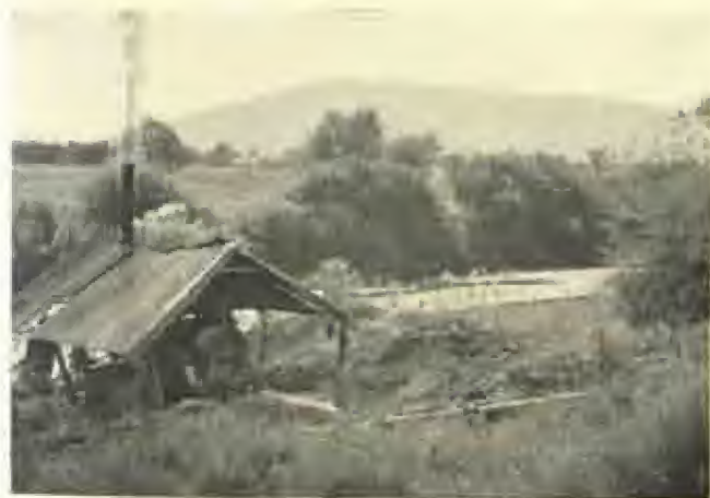
34. Pump for raising water from the Pienaars river in the Transvaal Bushveld Basin in order to irrigate wheat and tobacco lands. Except on the irrigation schemes this is the usual method of obtaining water for irrigation in the Bushveld. The photograph was taken in winter when the river carried very little water, the whitish patches being in fact stretches of sand in the river bed.
