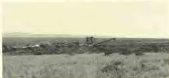
67. The Iscor iron ore workings at Tlhabazimbi. Situated on a hill about 1,000 feet above the general surface level, they consist of tunnels and open-face quarries. The man hoist (emphasized by the white dotted line), carries the miners to the main adit. A self-acting incline (emphasized by the black dotted line) laid diagonally across the hill-side is used for conveying the ore to the railhead.
