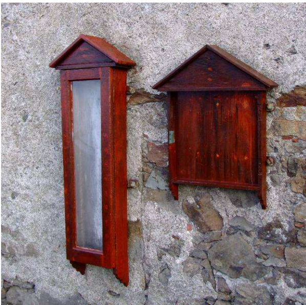
Banff Harbour Barometer Box & notice board partly refurbished. (Perspex fitted and varnished).
