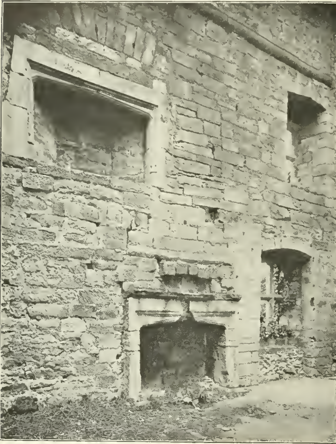
FIG. 2.—DILSTON TOWER. FIREPLACES ON FIRST AND SECOND FLOORS.
