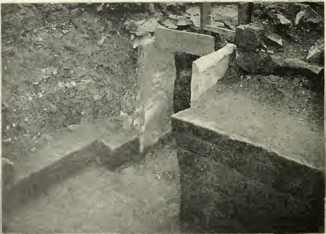
FIG. 12. VAULT IN SITE XLV (PRINCIPIA) SHEWING ENTRANCE FROM STEPS AND THE 'STEPPING' OF THE VAULT WALL TO FORM A ROOF.
