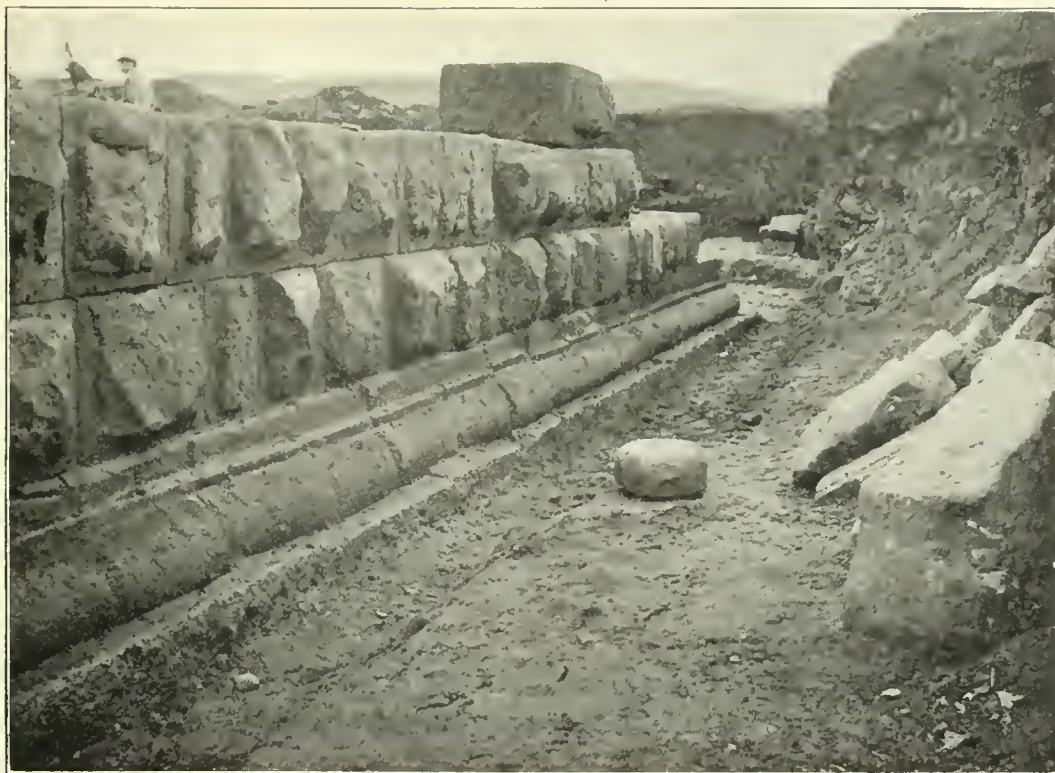
FIG. 6. VIEW OF WESTERN OUTER WALL OF SITE XI, SEEN FROM OUTSIDE, SHEWING PLINTH AND BOSSED MASONRY.
