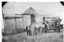
Log drying kiln built here and received lots of soft pine, spruce, fir and hemlock lumber. The kiln was built by the logging mill owned by Peter Peterson on his former logging farm on the same property the mill now occupies.
