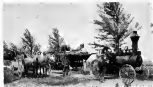
Threshing outfits moving from farm to farm often created traffic problems on the narrow roads common in McKelip only years ago. This threshing machine was operated by (l/r) John Deane, Mel Klene and Harry Deane. The picture was taken on the 12th of McKelip about 1918.
